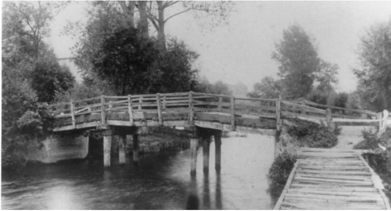
Dedham bridge in 1898, showing its central opening with three supporting posts on either side. On the right is the decking carrying the tow path across the tributary.
