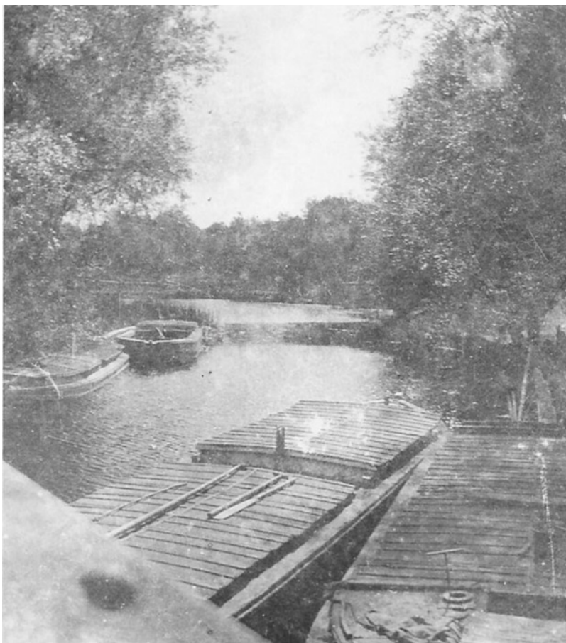
Ted Eley's photograph of barges parked up beside Dedham bridge (one of its rivets can be seen bottom left) in the early twentieth century. After they were introduced in 1705 bridges had to be altered to provide a wider central opening.
