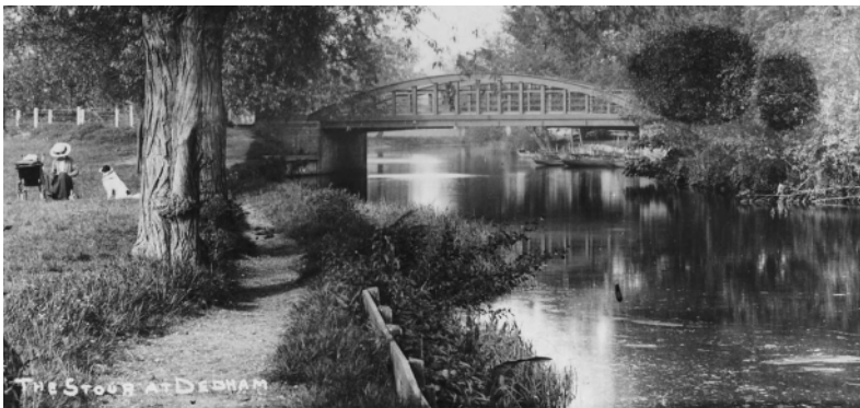
Dedham's iron bridge installed in 1900.
